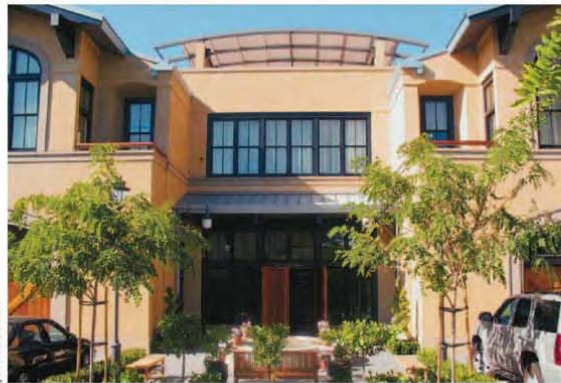
Berkeley's Design Review Committee was reportedly "knocked out" by Trachtenberg's plans for the elaborate mixed-use Read Building.
